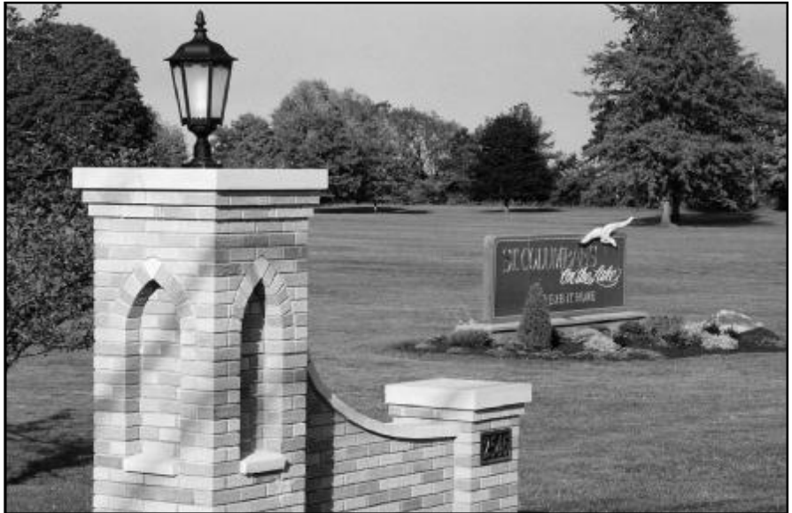
The renovated driveway entrance offers a graceful welcome to St. Columban's on the Lake Retirement Home.
